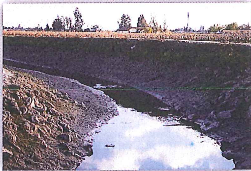
Figure 1 - Channels, streams, and drainage ways are over taxed by increases in runoff caused by increased development and impervious surfaces.
